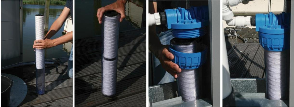
*Installing AC filter cartridges: 2 x 10" or 1 x 20" (transparent housing is only for picture)*
