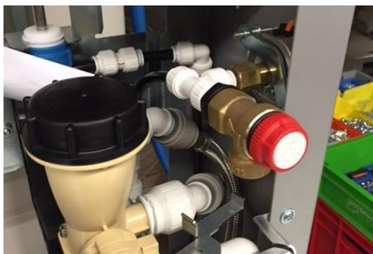
*Pressure relief Valve: in operation when pressure in the system exceeds 4 bar*
