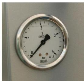
*Manometer, indicating the pressure of the Back Wash Buffer (collecting the water for the back wash)*
